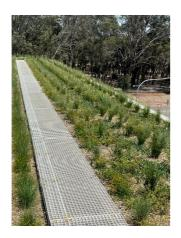
The Green Roof Mix has been developed to provide a stable substrate that can sustain plant life while maintaining volume over time.
